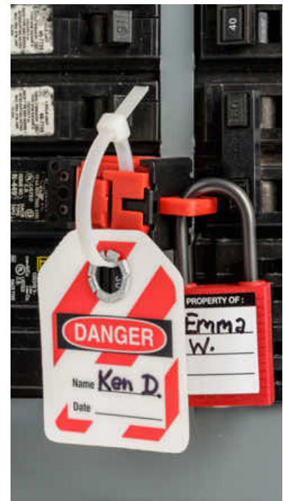
Can be secured with cable ties and/or a safety lock
